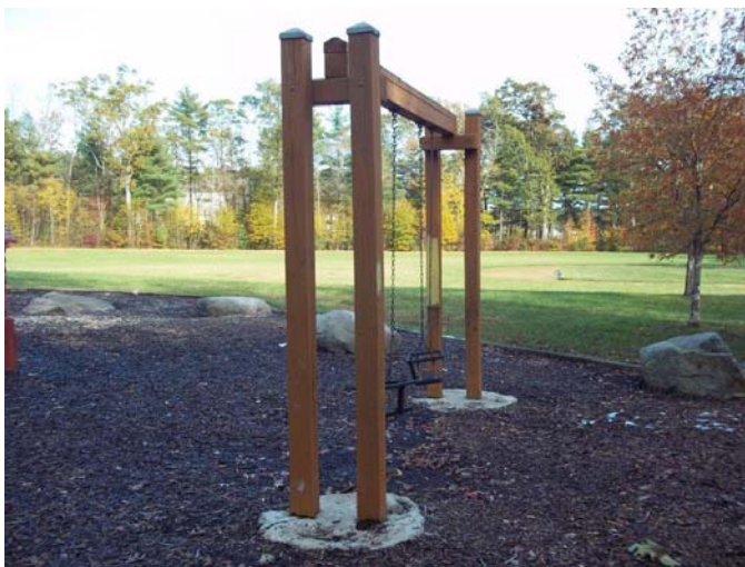
Exposed Concrete Footings, Rusty Swing Chains, & Worn Out Swing Seats.
